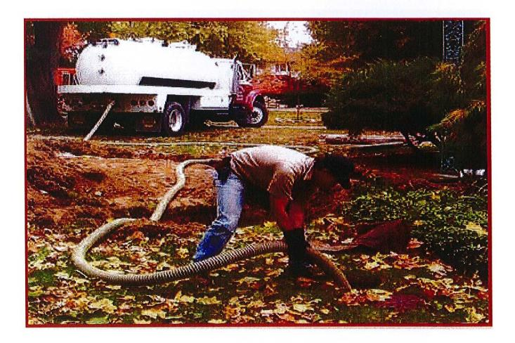
What will happen if on-lot septic systems are not properly operated and maintained? The system may fail contaminating groundwater and water supply wells, creating health hazards.
