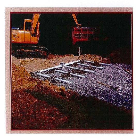
Clear waste water flows through the aggregate and into the **suitable soil (soil)**.
